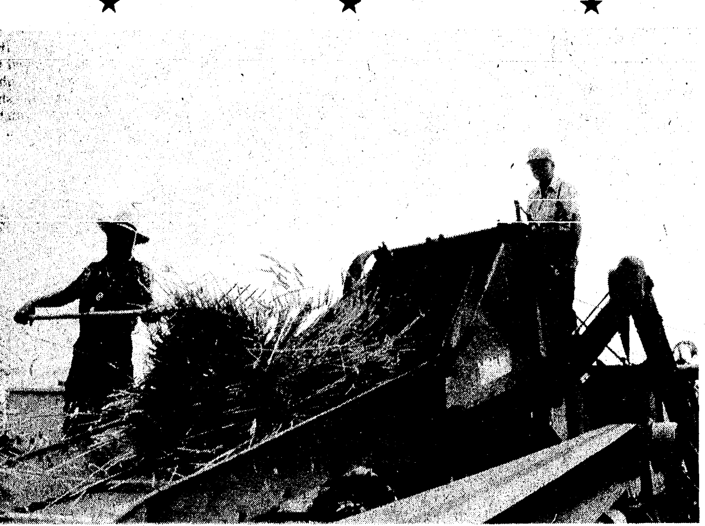
CORN STALKS have to be shredded before going into a silo, and this antique machine formerly was used to do it. The same technique to make silage is still employed, but the equipment is more modern.
