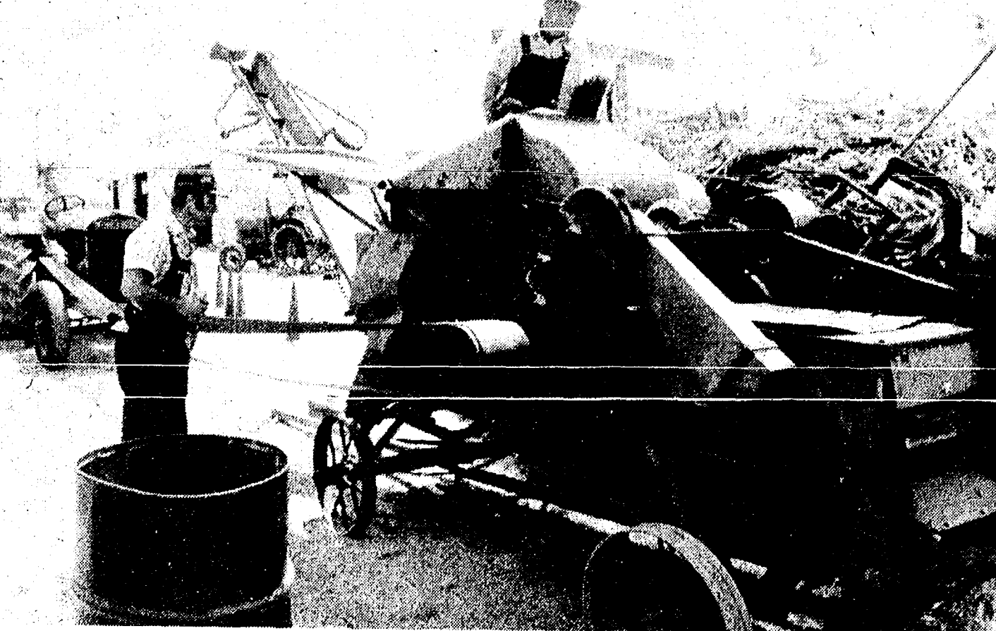
CORN STALKS have to be shredded before going into a silo, and this antique machine formerly was used to do it. The same technique to make silage is still employed, but the equipment is more modern.
